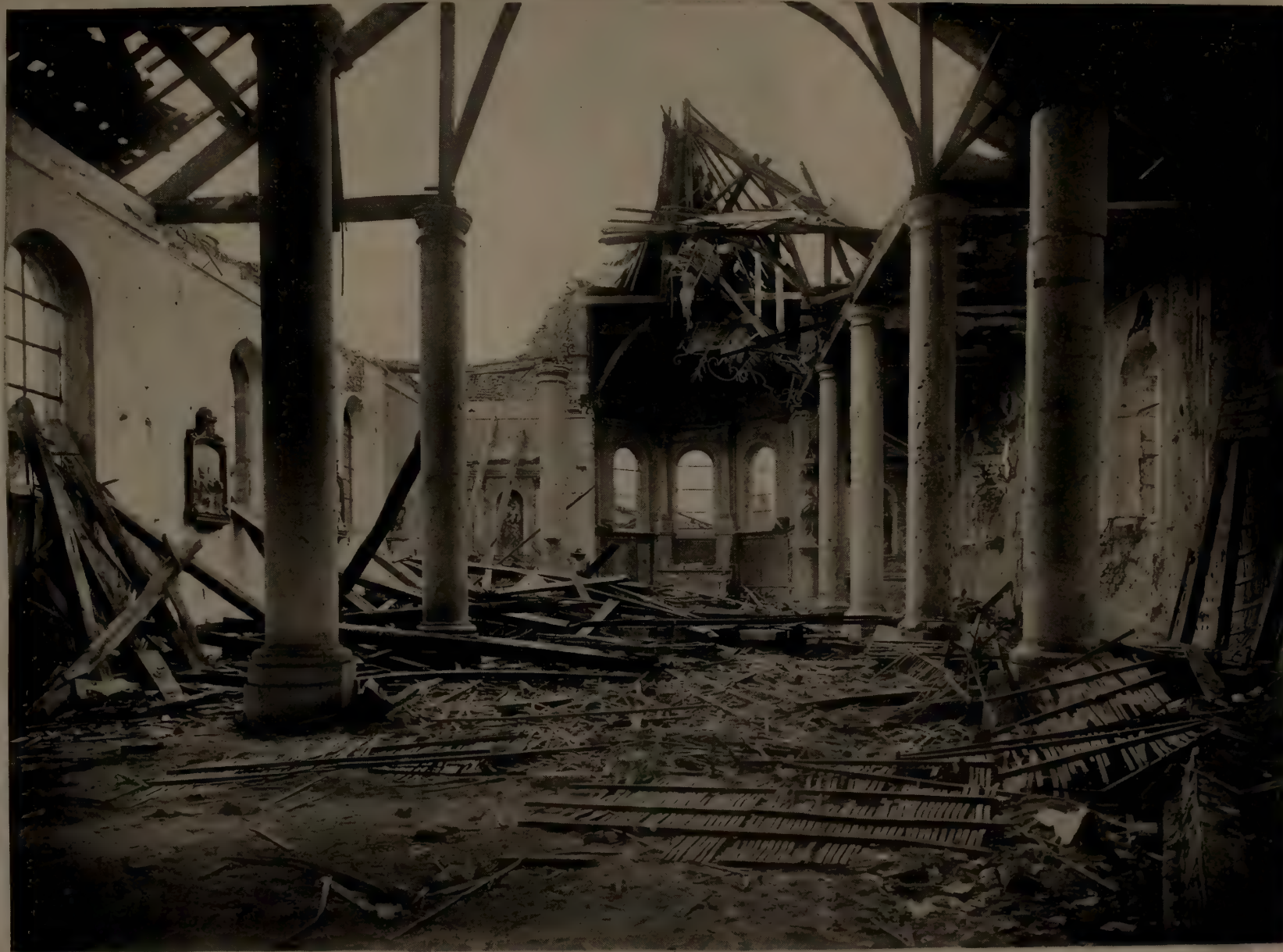
Wrecked Church at "Sivry"
